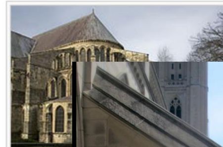
Early flying buttress on the eastern apse of Remi in Reims.
